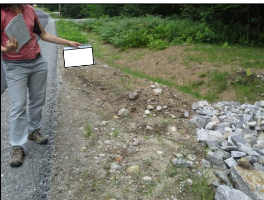
After — Town road site after the road work was completed. As shown in the picture to the left, the road shoulder is still slightly unstable, rendering the site a low impact, rather than a no impact site. The new culvert is larger and its ends have been stabilized with stone.
