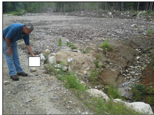
This high impact logging site was a large area that flowed under the access road via a culvert and then directly into a stream. This site was atypical of logging sites, in that there were not that many landings documented.
