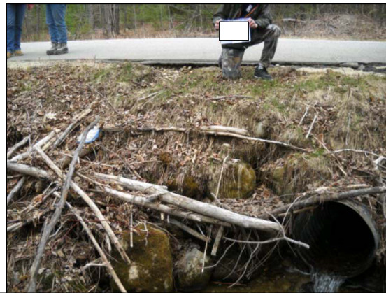
Before - This Roxbury town road site originally ranked as high impact with moderate road surface erosion, several road shoulder erosion and winter sand deposition into the stream.
