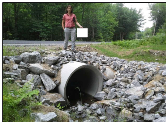
After — Town road site after the road work was completed. As shown in the picture to the left, the road shoulder is still slightly unstable, rendering the site a low impact, rather than a no impact site. The new culvert is larger and its ends have been stabilized with stone.
